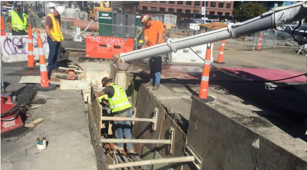
Example of underground electric utility installation.
